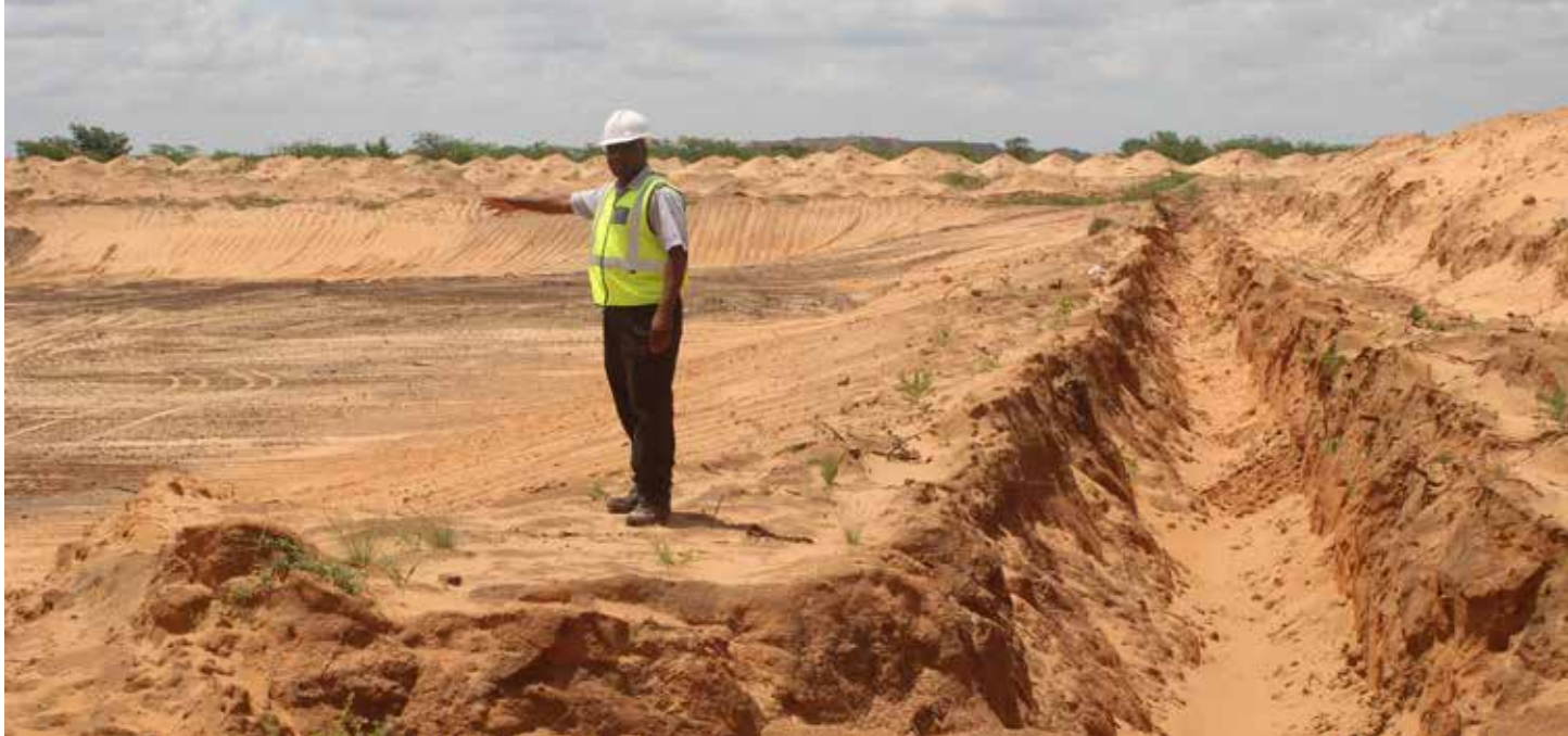
TOP SOIL STRIPPING AHEAD OF FUTURE DEVELOPMENT OF LANDFILL
