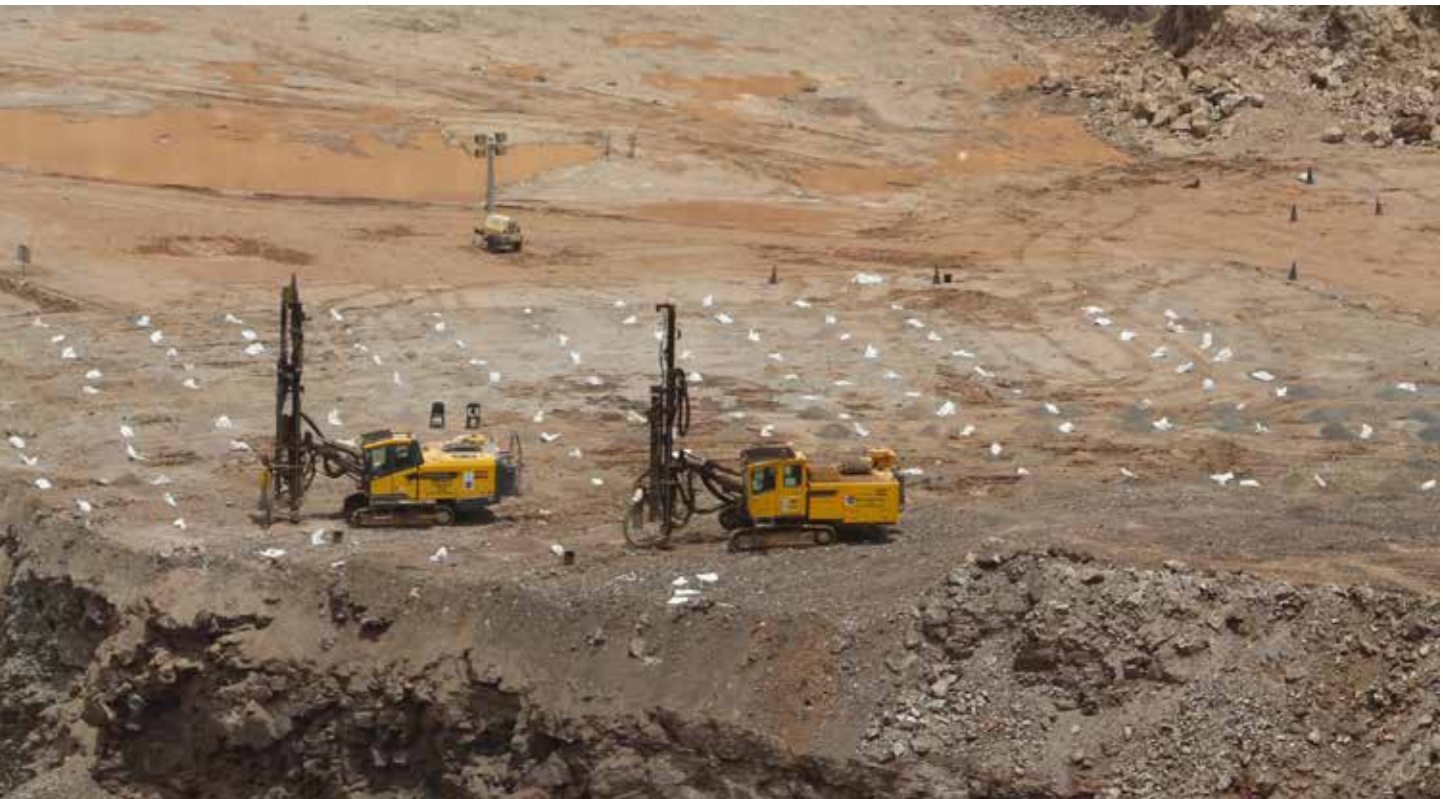
RIGS DRILLING A SERIES OF BLAST HOLES AT KAROWE
