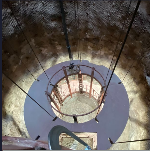
Vent Shaft Pre-sink stage view from above
