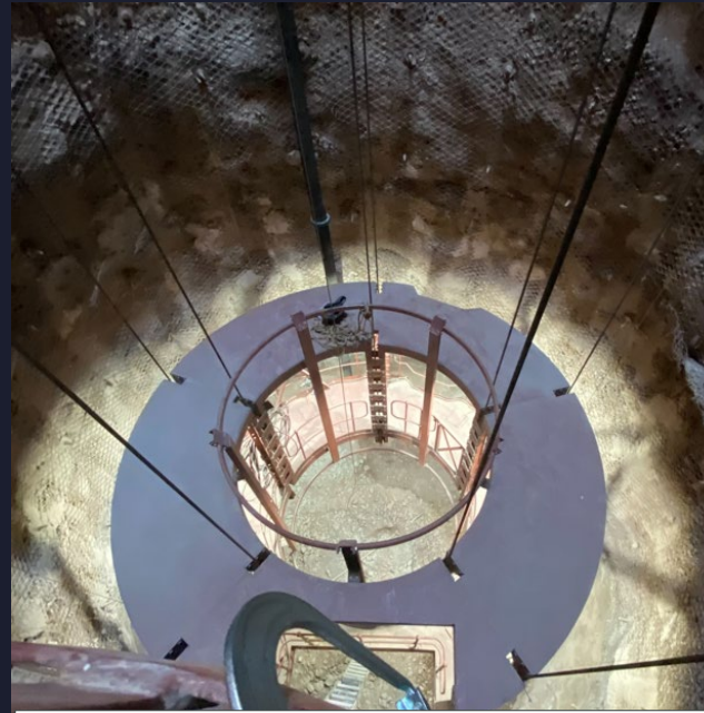
Vent Shaft Pre-sink stage view from above
